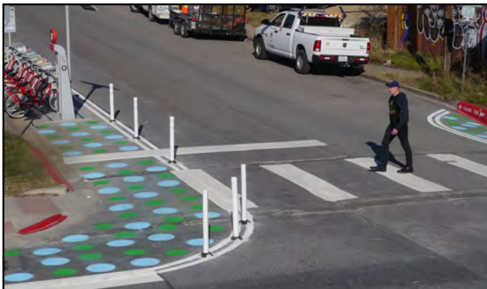
Painted pedestrian bulb-outs (with installed barriers) can be a cost-effective way to increase safety and visibility at an intersection.
