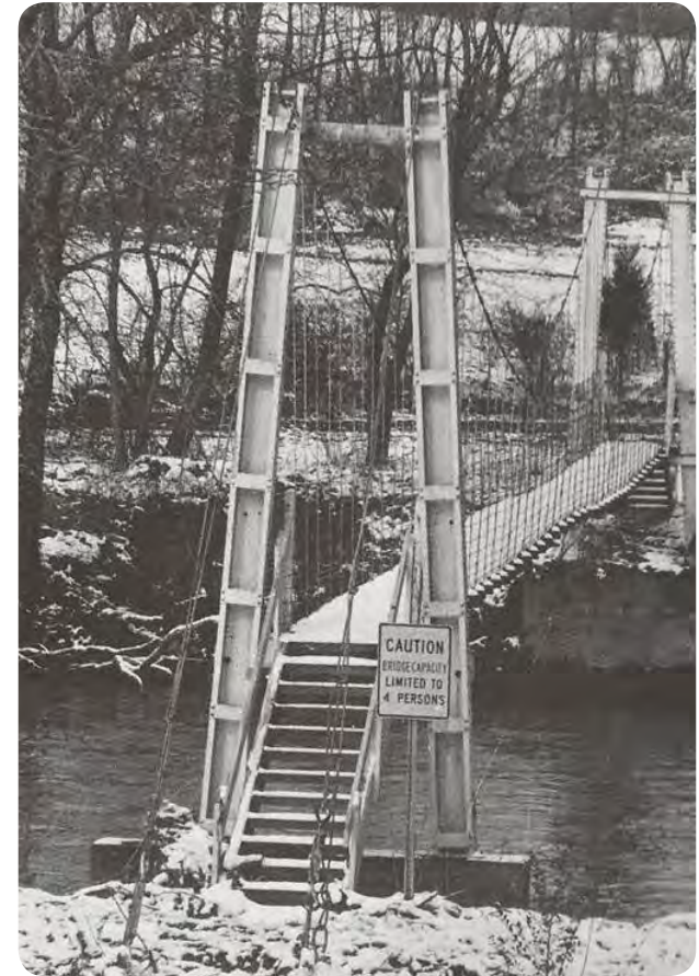
Macon County residents have a history of walking. "The North Carolina Department of Transportation built pedestrian suspension bridges to give rural residents a quick way on foot across a major river. This one, which crosses the Little Tennessee River in the Etna Community, had to be rebuilt after it was destroyed by flood." - NC Study List
